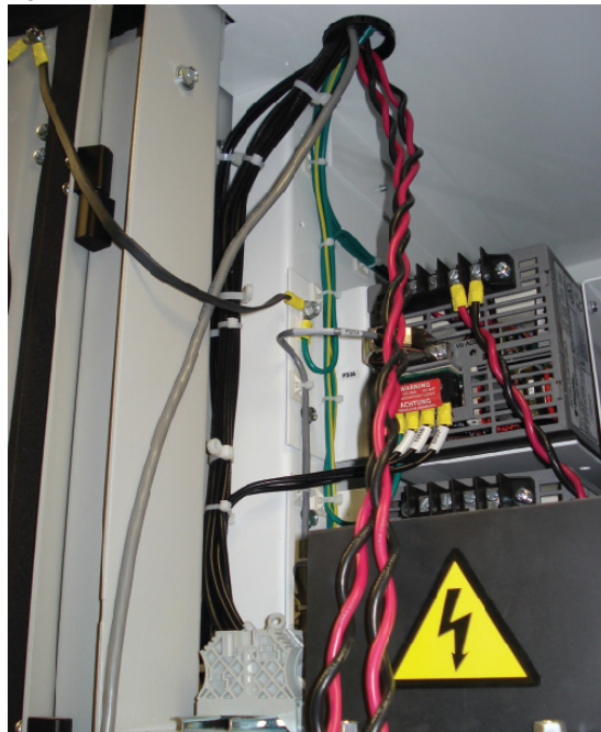
Figure 33 - Belden Shielded Cables
