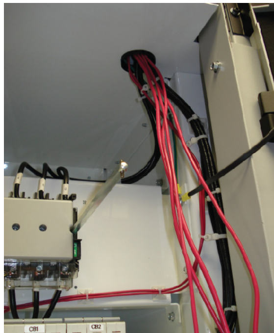
Figure 35 - Route Control Wires through Grommeted Cutout
