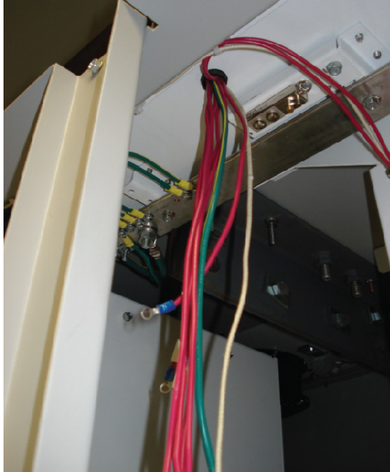
Figure 34 - Fan Thermostat Control Wires
