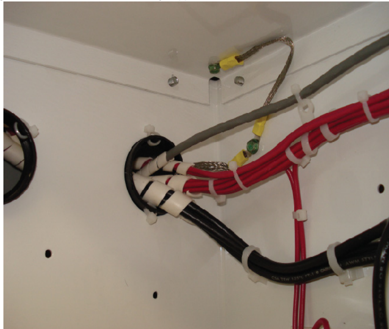
Figure 40 - 120V and XIO Cables through Upper Cutout
